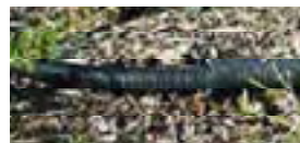
Above: Perforated hose is attached to the greywater system and run around the well-mulched garden. These pipes should be laid below the surface at a 2% slope (2cm drop per metre) to provide the safest way of using greywater, a more efficient way to irrigate and reduces evaporation.
