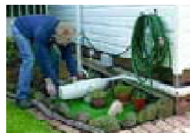
Above: All water from the shower and the laundry is piped into a greywater system, which returns it to the toilet cistern for flushing.
