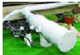
Above: The capacity of this system is about 150 litres. What isn't used in the toilet is pumped automatically onto the garden once daily.
